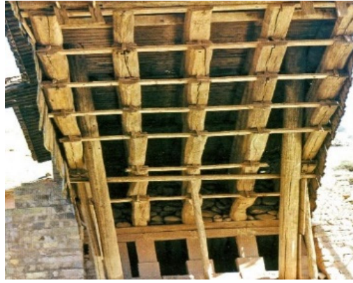
Fig 4. Tongjing Bridge single outrigger beam system pick out 7 times
