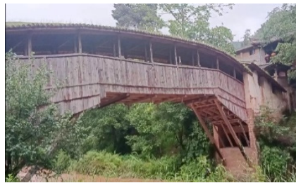
Fig 7. Yunlong County Caifeng Bridge gallery at both ends of the building archway or bridge pavilion
