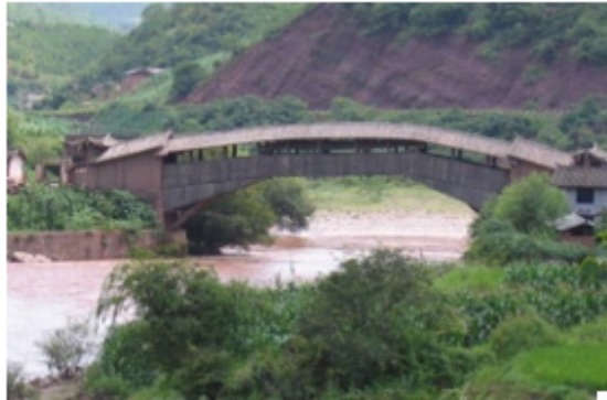
Fig 2. Bridge piers are set at both ends of Tongjing Bridge
