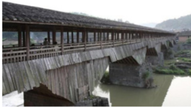
Fig 3. Five ship-shaped stone piers are erected in the middle span of Wan' an Bridge
