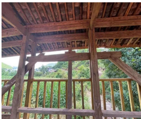
Fig 6. Yonglai Bridge internal saddle frame system
