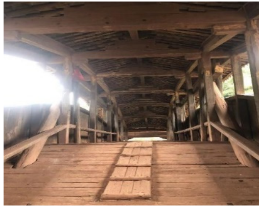
Fig 5. Internal structure of saddle frame system
