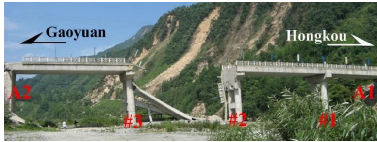
(a) The collapse of Gaoyuan bridge
