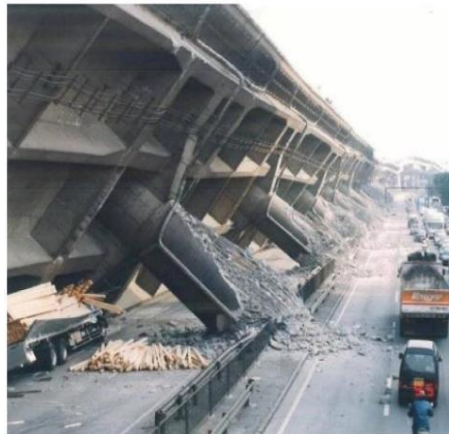
(b) Post-seismic photo of the collapsed bridge
