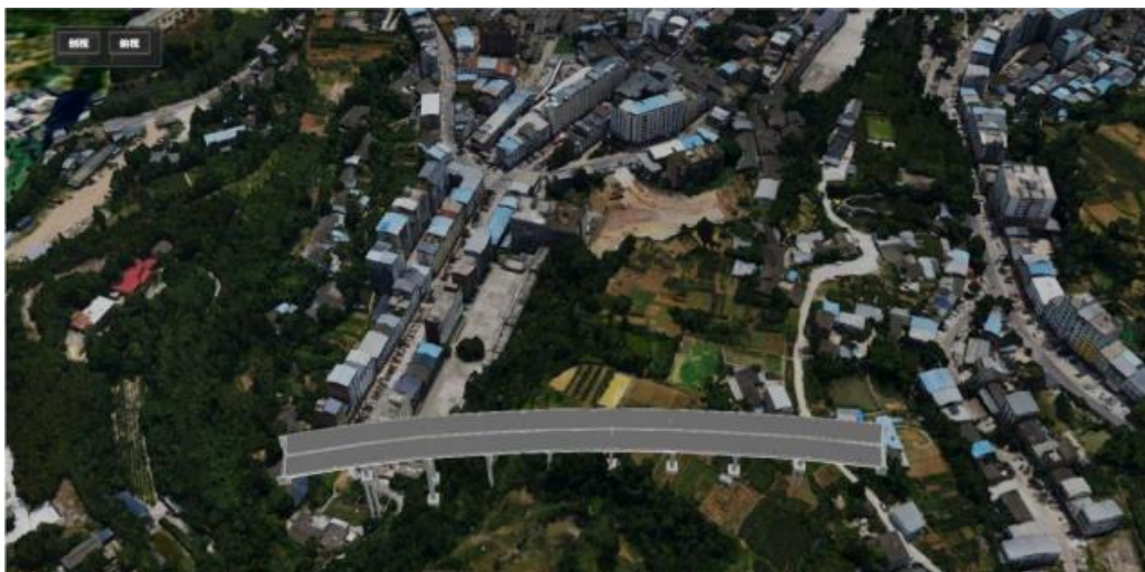
Figure 1. Side view of the bridge [3]
