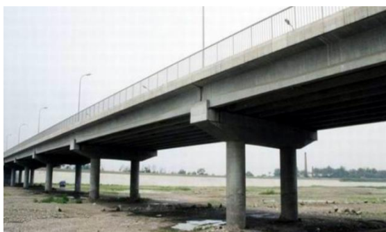
(a) Bridge structure in 2013
