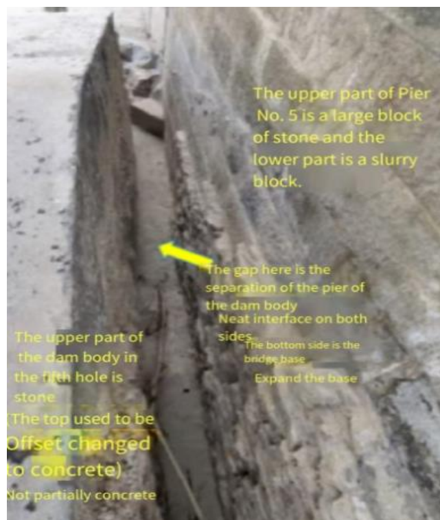
Figure 8. Structural Components and Modifications of Pier No.5 [8]
