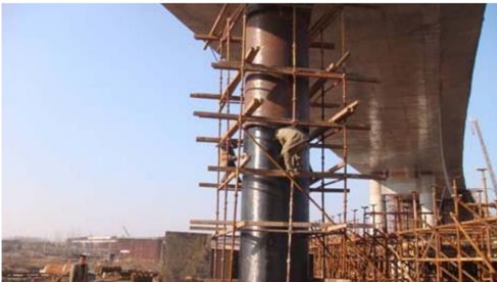
Figure 1. The process of FRP pasting of the concrete filled FRP-steel composite tube pier for Chengqiao hinge [13]
