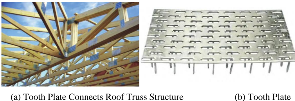
Figure 2. Tooth Plate Connection Joint [4]
