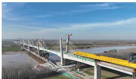
Figure 1. Changqing Yellow River Bridge [8]
