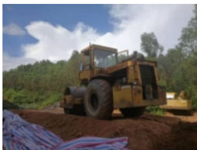
Fig1. The test earth embankment preparation
