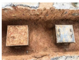
Fig3. Shear box installation
