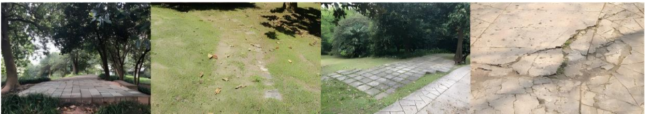
Fig. 5. Current status of site roads and paving
