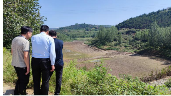
Fig. 2 Reservoir Condition After Water Drainage
