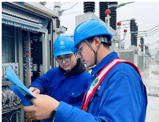
Figure 2. Ultra-high voltage equipment maintenance
