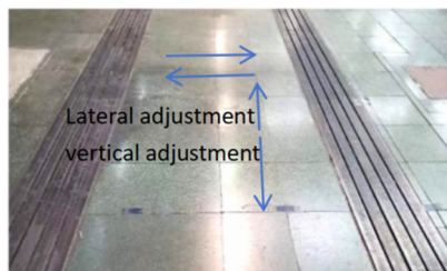
Figure 4. Pre-buried I-beam assembly
