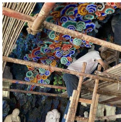
Figure 2 Photo of the Buddha Statue Construction Project at Guanyin Temple in Baotou City
